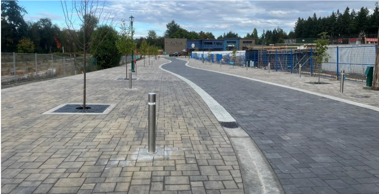
Woonerf currently under construction on 2 nd Avenue in Qualicum Beach
