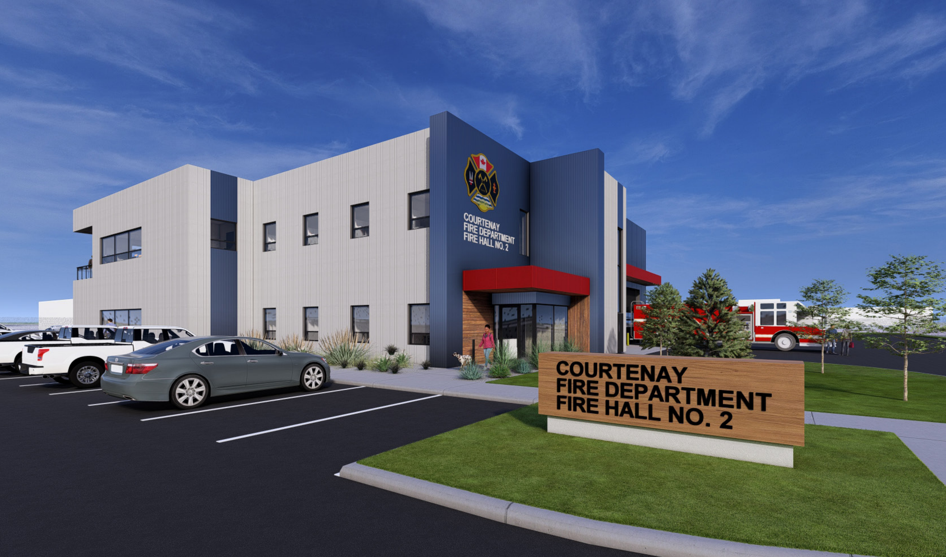
Courtenay Fire Hall No.2
