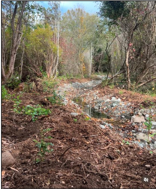
Figure 5: DPA-4 - 4694 Headquarters - Site Photos as built
