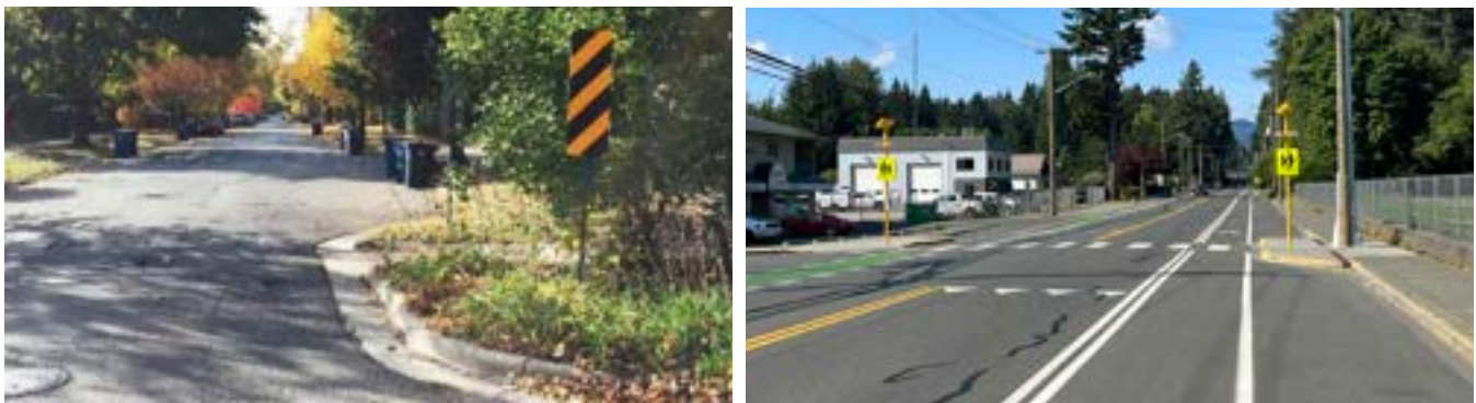
Figure 12. Sample Application of Curb Bulge 18, 19
