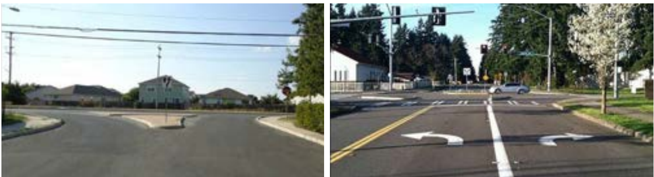
Figure 20. Sample Application of Forced Turn Island 30, 31
