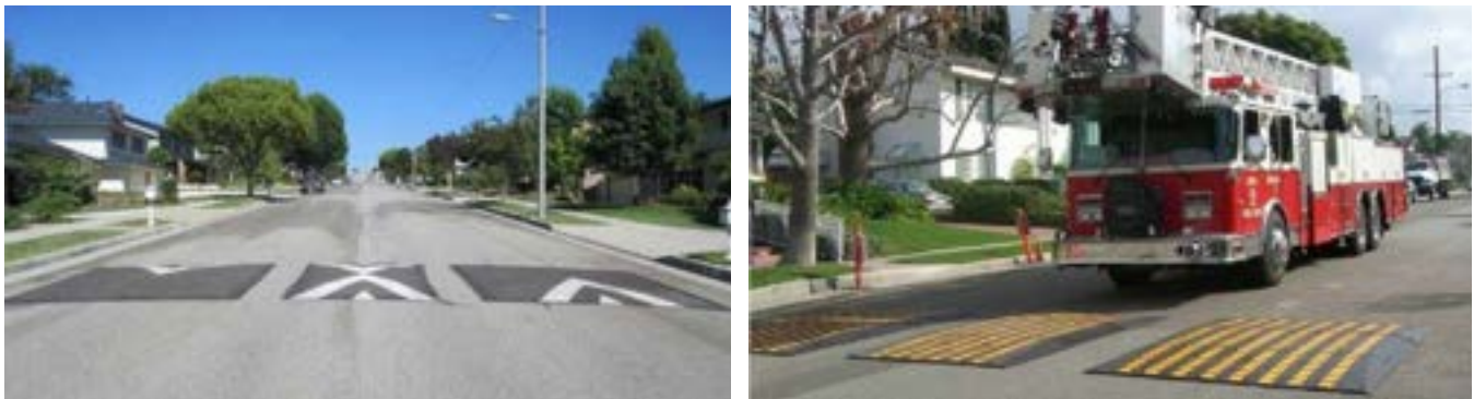
Figure 8. Sample Application of Speed Cushion 12
