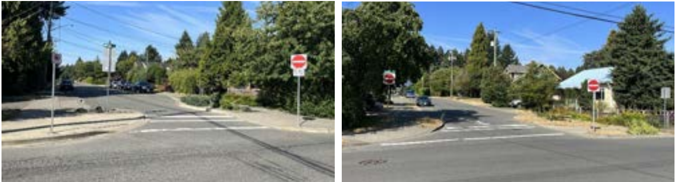
Figure 16. Sample Application of Half Street Closure 25, 26
