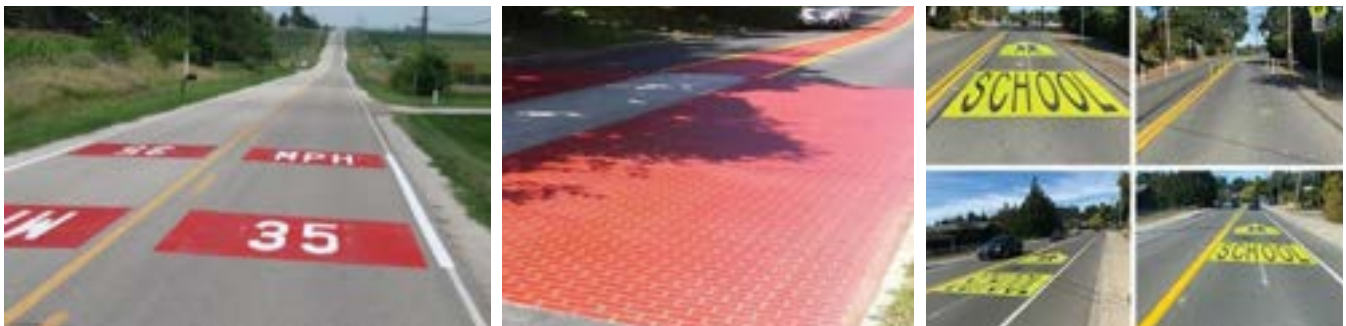
Figure 24. Sample Application of Surface Treatments 39, 40, 41
