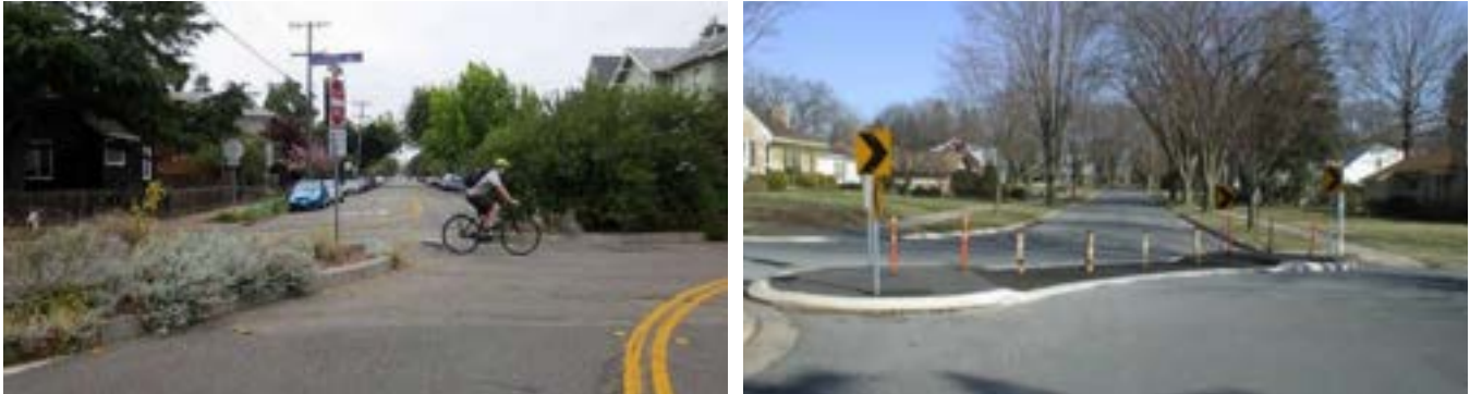
Figure 18. Sample Application of Diagonal Diverter 27, 28
