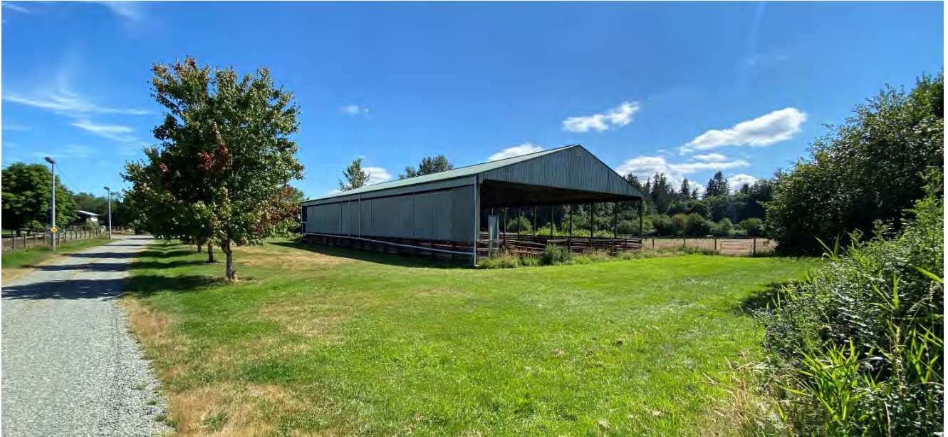
Site Photo 14: Zone G - Stonehenge Farm Expansion. South-east view from tree-lined Dove Creek Place entrance (with existing covered riding ring on right).
