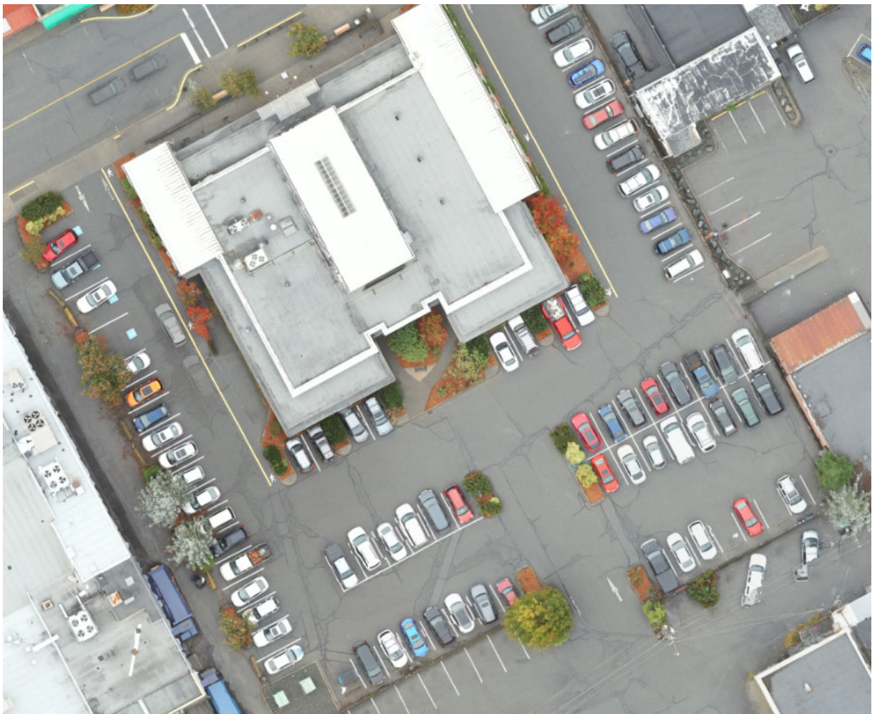
Figure 19: Vancouver Island Public Library parking lot
