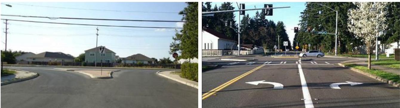
Figure 20. Sample Application of Forced Turn Island<sup>30, 31</sup>
