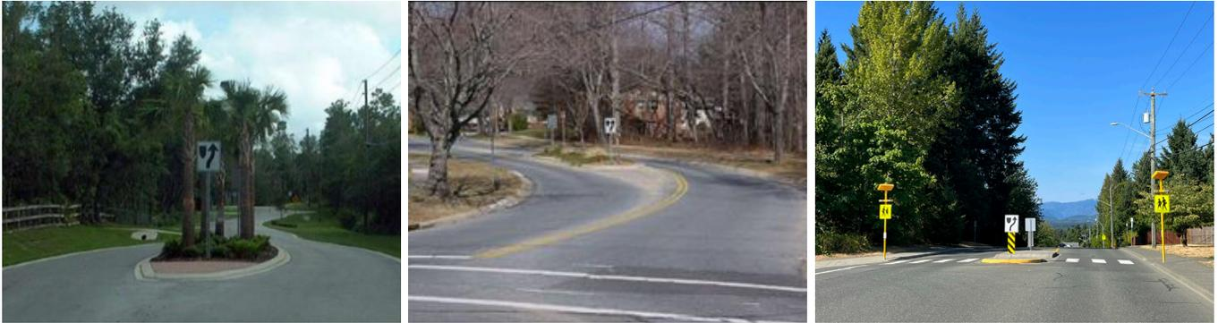
Figure 13. Sample Application of Median Island (Mid-Block – Left, Neighbourhood Entrance – Middle, With Crosswalk – Right)<sup>20, 21</sup>
