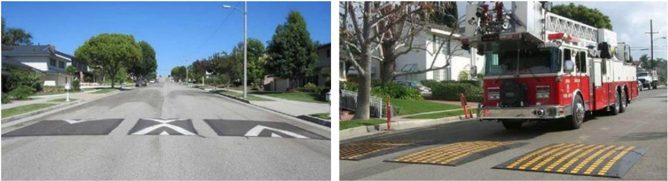
Figure 8. Sample Application of Speed Cushion<sup>12</sup>
