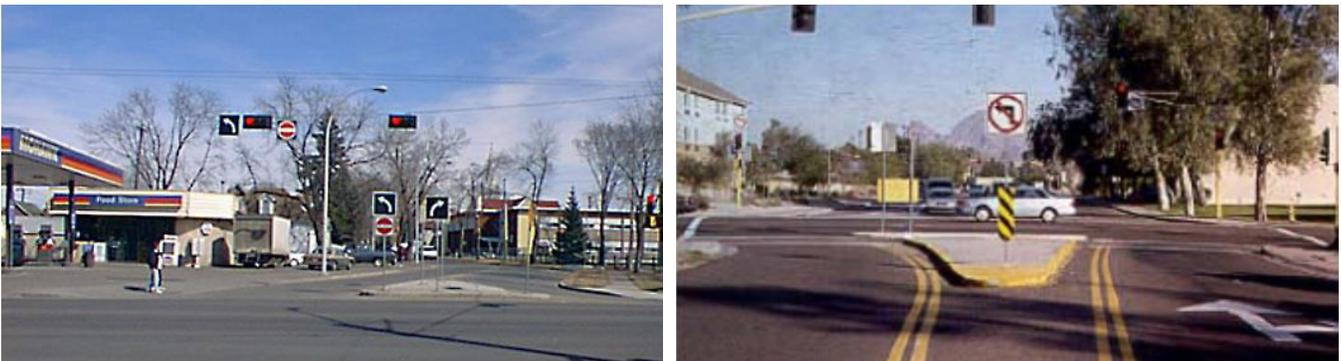
Figure 21. Sample Application of Intersection Channelization<sup>32, 33</sup>
