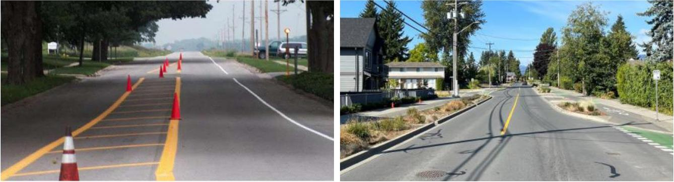
Figure 14. Sample Application of Lane Narrowing<sup>22, 23</sup>
