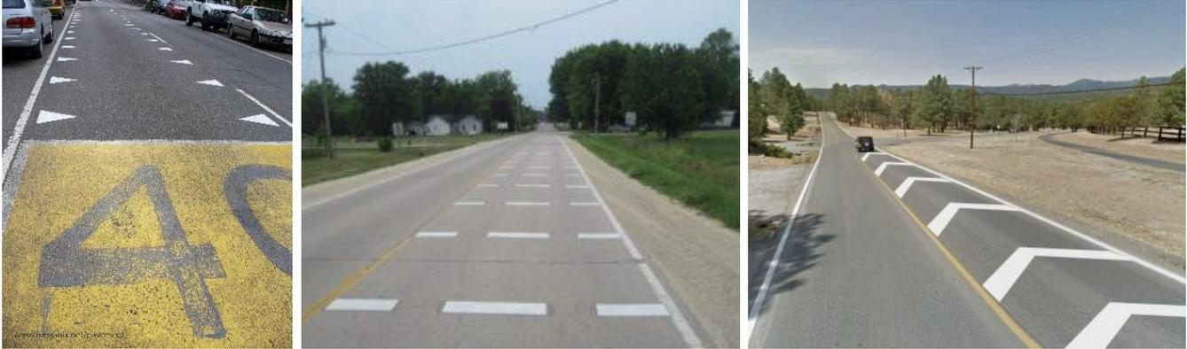
Figure 23. Sample Application of Transverse Lane Markings (Dragon Teeth – Left<sup>36</sup>, Transverse Bars<sup>37</sup> – Middle, Converging Chevrons<sup>38</sup> – Right)
