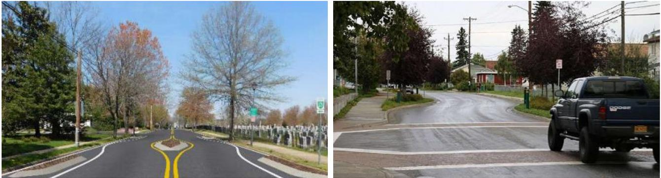
Figure 1. Sample Application of Chicane<sup>1, 2</sup>
