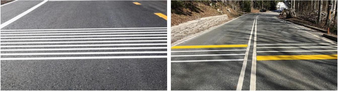
Figure 25. Sample Application of Rumble Strips<sup>42, 43</sup>
