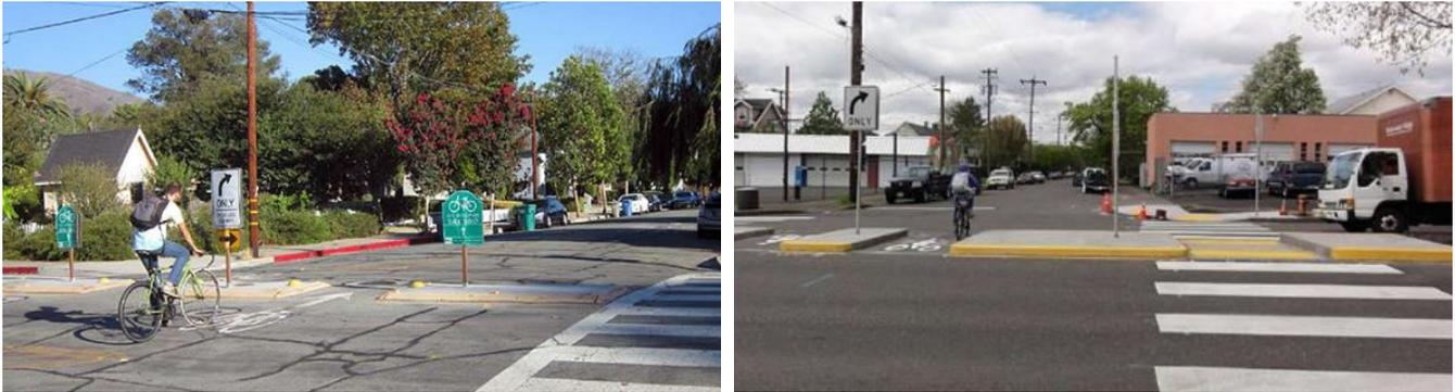
Figure 19. Sample Application of Median Barrier<sup>29</sup>
