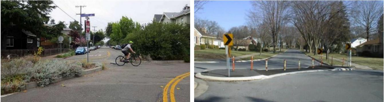
Figure 18. Sample Application of Diagonal Diverter<sup>27, 28</sup>
