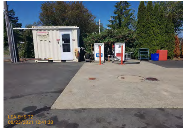
Fueling tank area viewed to the northwest
