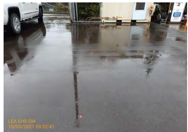
Utility line location points near the fueling tank area
