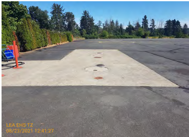
Fueling tanks area viewed to the northeast
