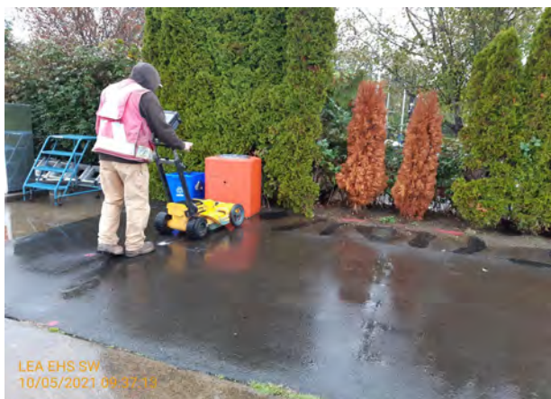
Utility locate scans near the fueling tank area
