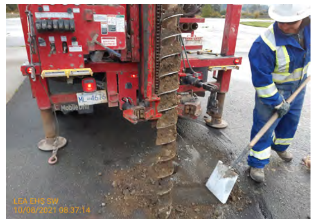
Solid stem auger borehole drilling
