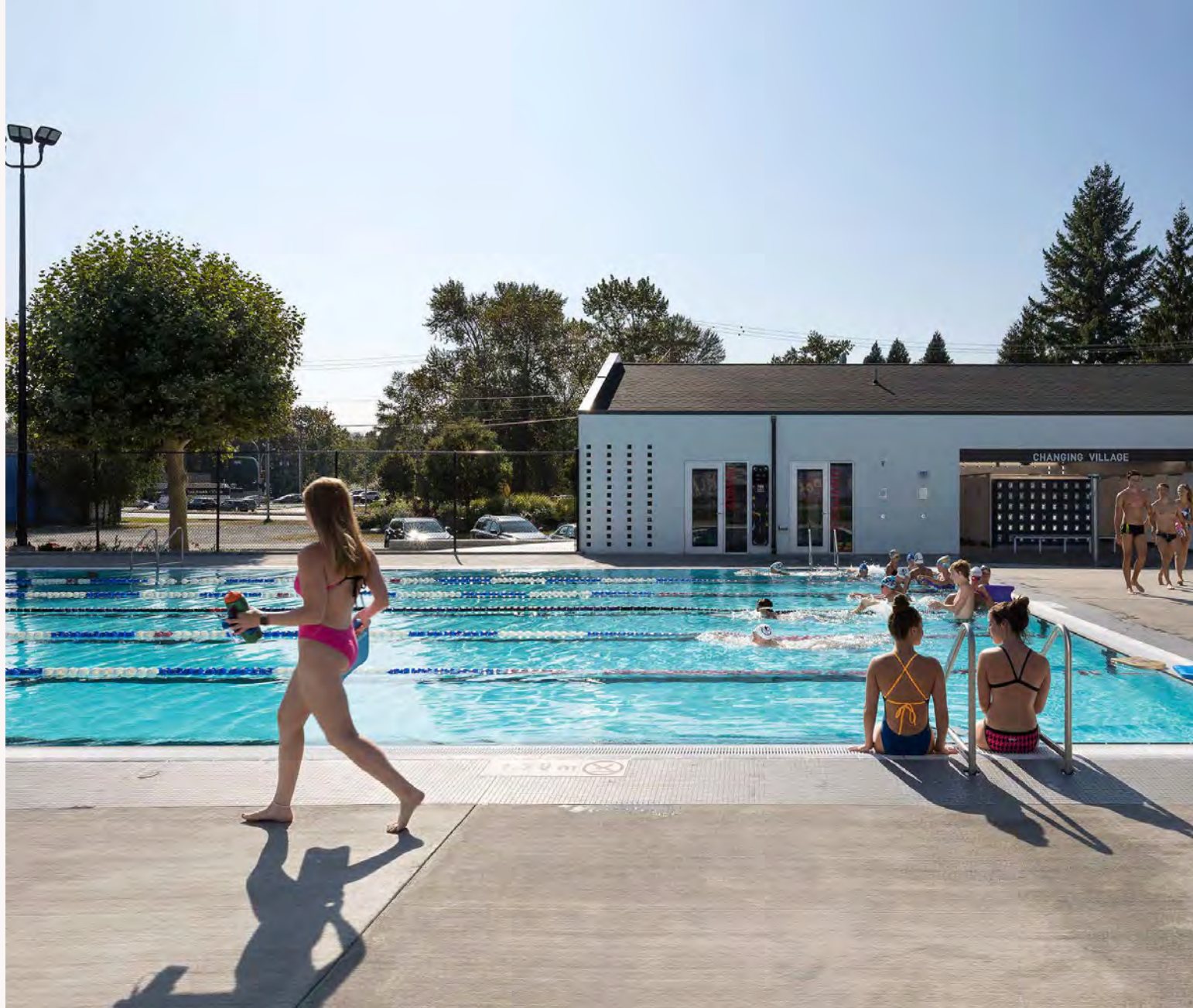
Centennial Pool Rehabilitation (2019) City of Port Coquitlam
