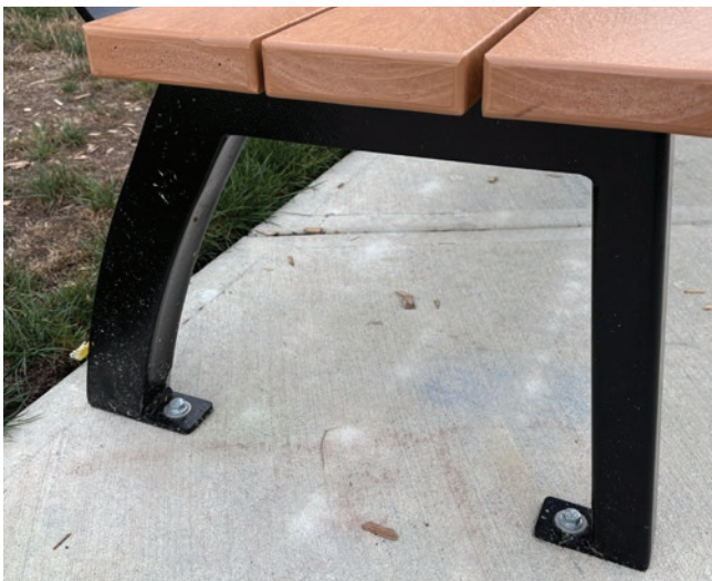
A surface mounted bench in a hardscape setting.
