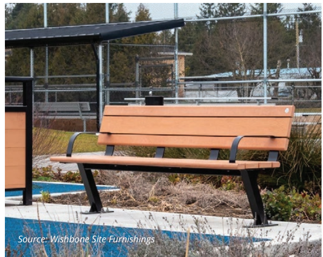
A poured-in-place concrete pad provided for a bench installation.
