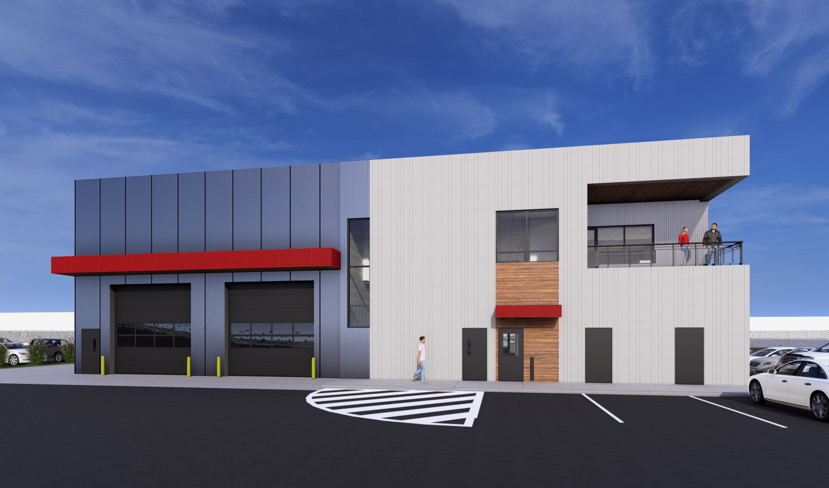
Courtenay Fire Hall No.2
