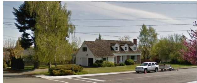
Figure 1: View of Subject Property at 1814 Grieve Ave
