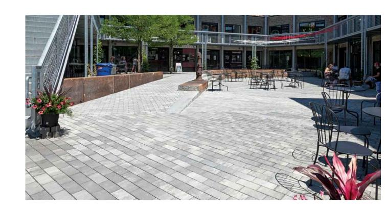
PERMEABLE PAVERS: ECO-PRIORA STANDARD PAVER RUNNING BOND PATTERN; PROVIDE COLOUR SAMPLE, TBD BY OWNER; OR SIMILAR, TO BE PREAPPROVED BY OWNER. INSTALL TO MEET ICPI & MANUFACTURER'S SPECIFICATIONS.
