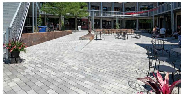
PERMEABLE PAVERS: ECO-PRIORA STANDARD PAVER RUNNING BOND PATTERN; PROVIDE COLOUR SAMPLE, TBD BY OWNER; OR SIMILAR, TO BE PREAPPROVED BY OWNER. INSTALL TO MEET ICPI & MANUFACTURER'S SPECIFICATIONS.
