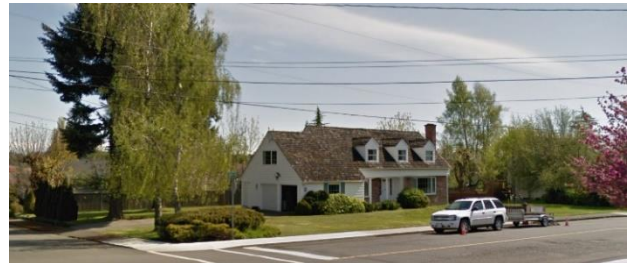
Figure 1: View of Subject Property at 1814 Grieve Ave
