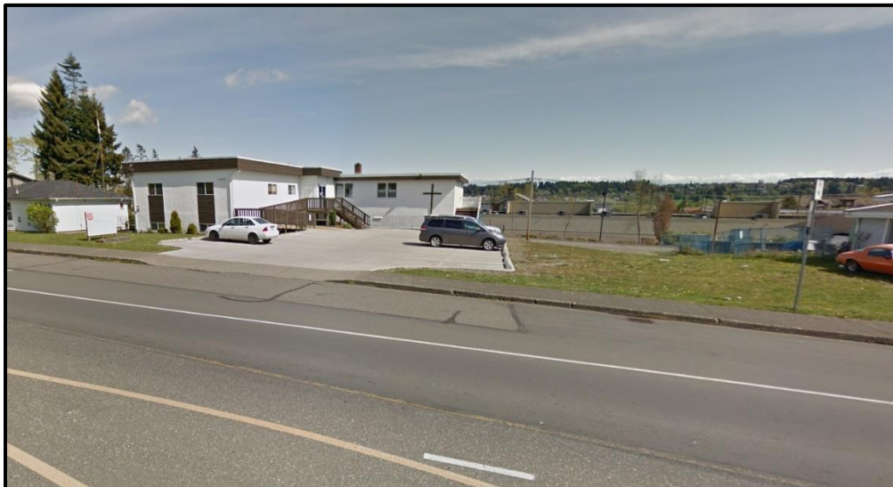
Figure 3: Existing Site from Fitzgerald Avenue
