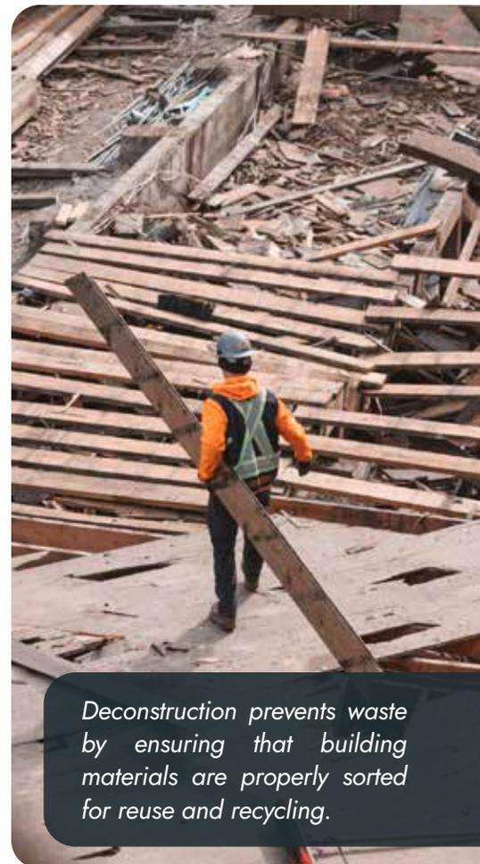
*Deconstruction prevents waste by ensuring that building materials are properly sorted for reuse and recycling.*
