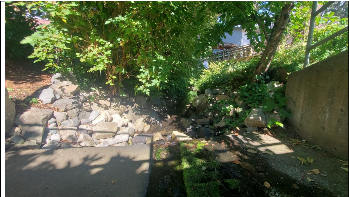
Photo 4. View downstream taken from the culvert headwall apron at the outlet of the culvert under 12 th St. E within the City SRW showing low flow conditions and bank armouring. The subject property is at left of image.
