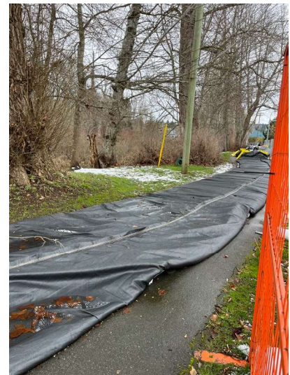
Figure 6-30: Deflated Aquadam (Credit: Ebbwater, 27 Feb 2023).
