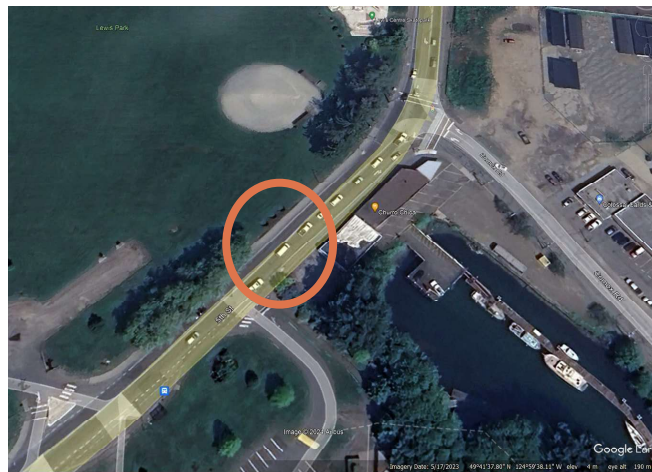
Figure 6-32: Lewis Park Culverts, connecting Lewis Park to Courtenay Slough. (Credit: Google Earth Imagery, 17 May 2023).
