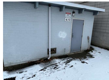
Figure 6-19: Anderton lift station, with the outside vent visible.
