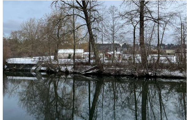
Figure 6-26: Lewis Park Dike, viewed from the west shore of the Courtenay River (Anderton Ave area). (Credit: Ebbwater, 27 Feb 2023).
