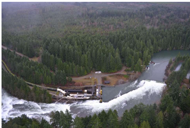
Figure 6-11: Dam Spillover during the 2014 flood at the Puntledge Diversion Dam (Photo credit: City of Courtenay).
