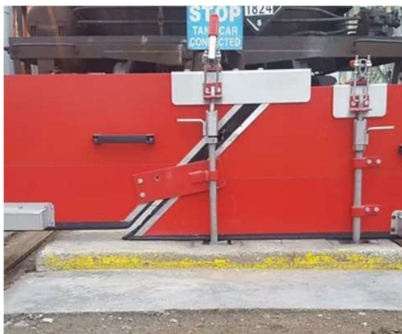
Figure 7-8: Chemical containment barrier (Credit: Flood Control Canada).
