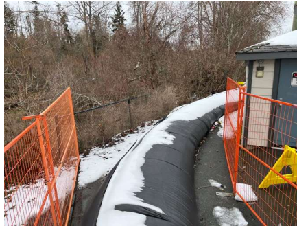
Figure 6-29: Aquadam near Lewis Park (Credit: Ebbwater, 27 Feb 2023).
