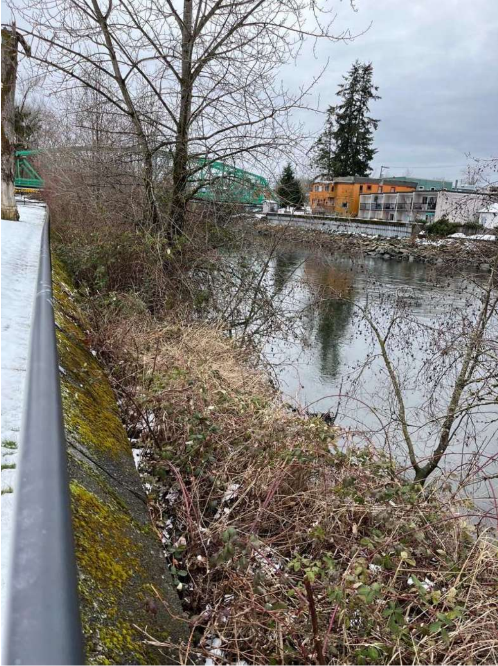
Photo 13: Vegetation along the toe and face of the Lewis Park Dike.
