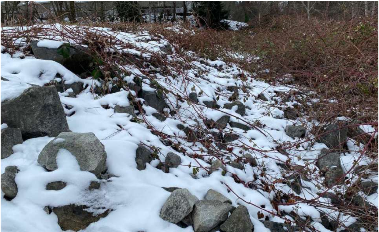
Photo 15: Riprap on the riverside of the Condensory Dike.
