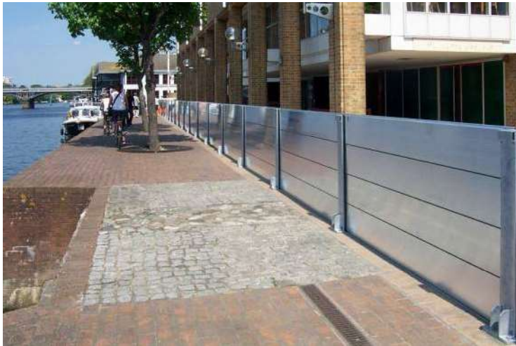
Figure 7-2: Stop Log Barrier (Flood Control International, 2023)
