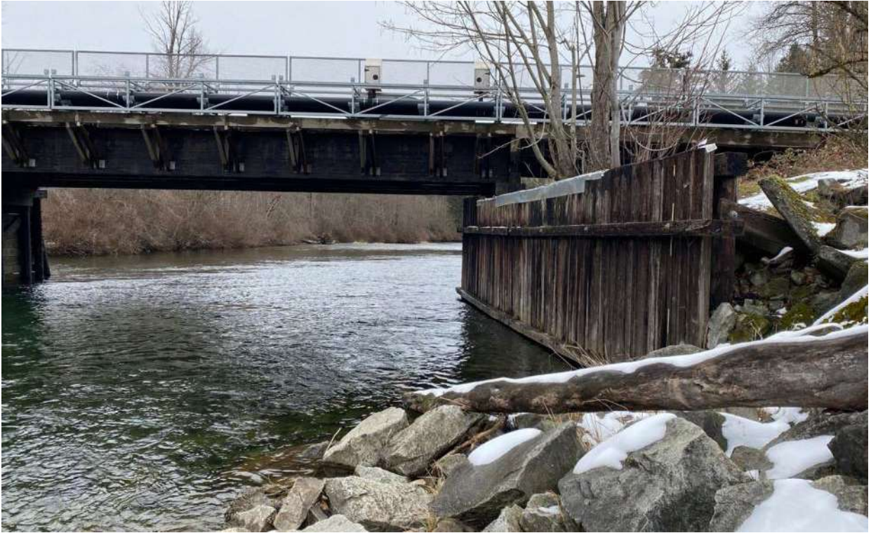
Photo 17: Condensory Bridge at downstream end of the Condensory Dike.
