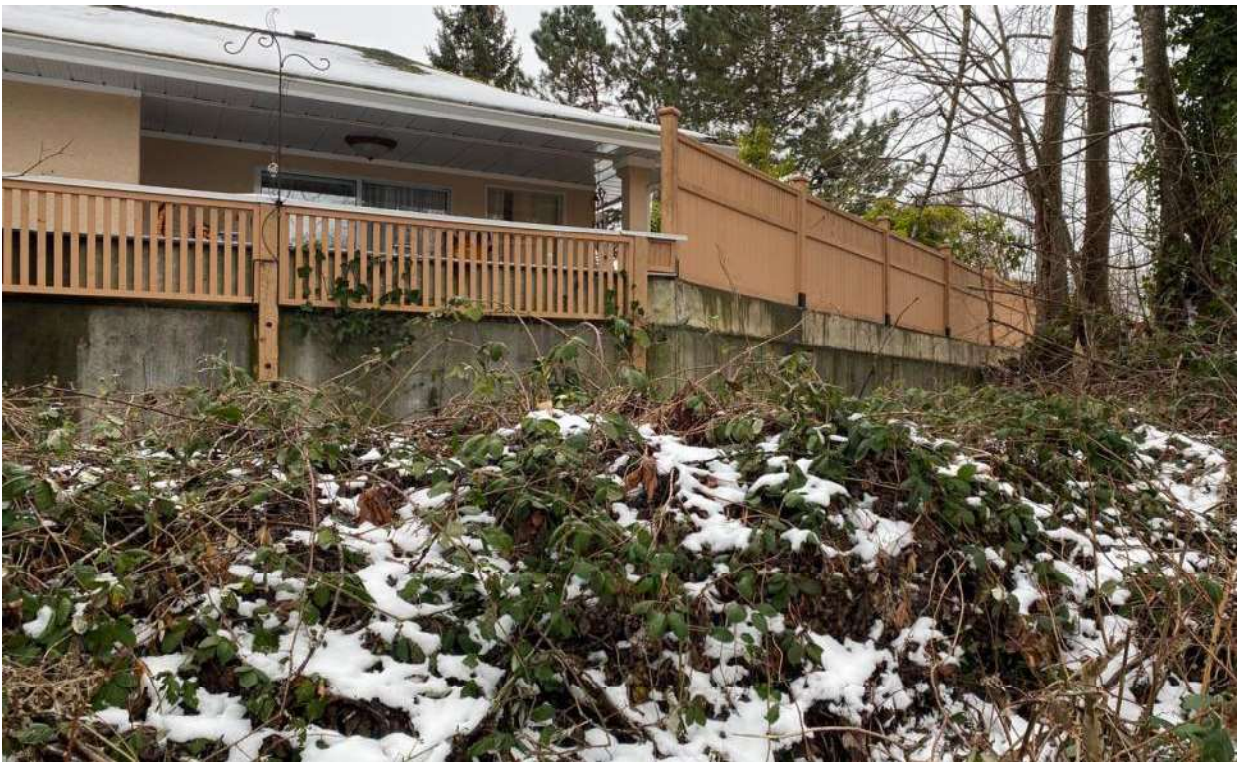
Photo 19: Canterbury Lane Dike with setback concrete wall and vegetation visible.
