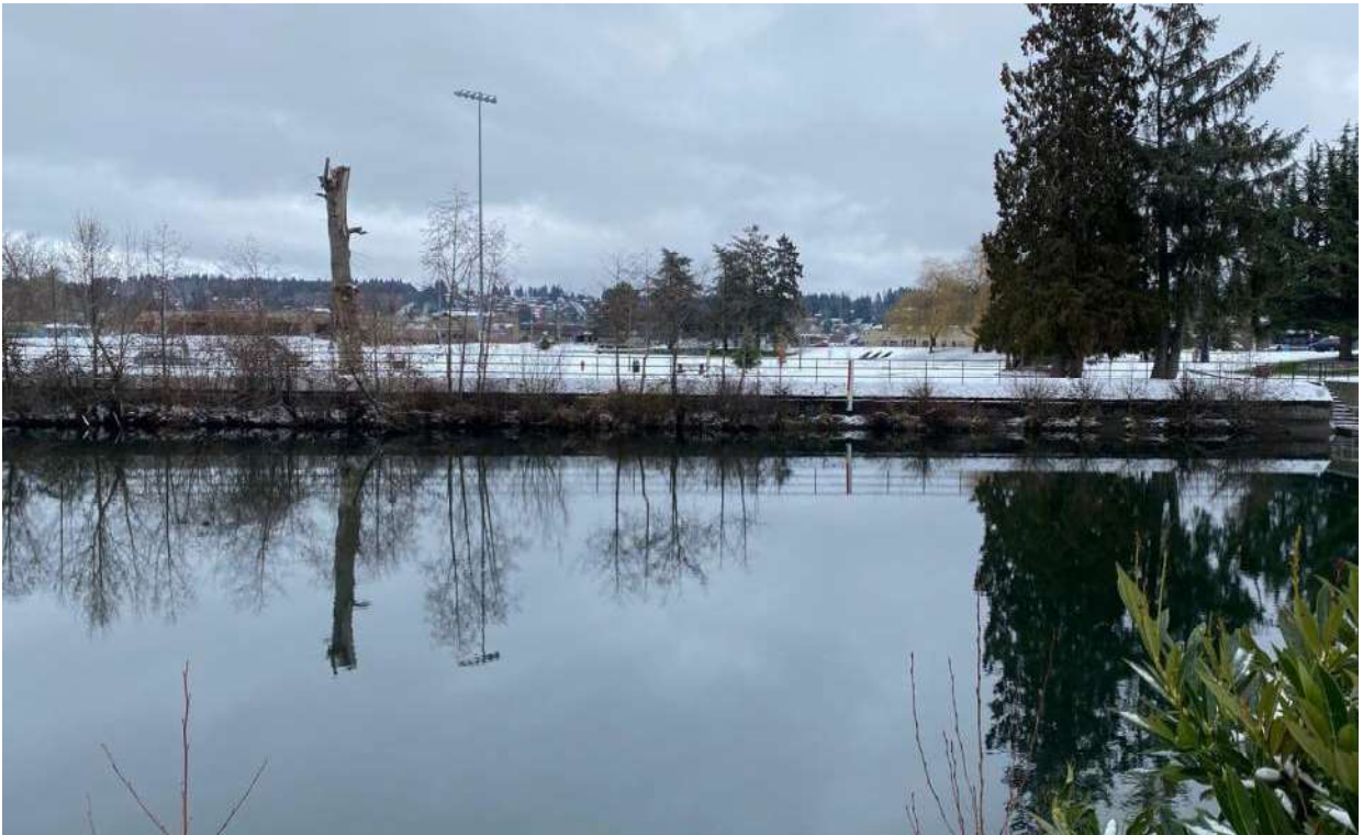
Photo 7: Lewis Park Dike concrete retaining wall.
