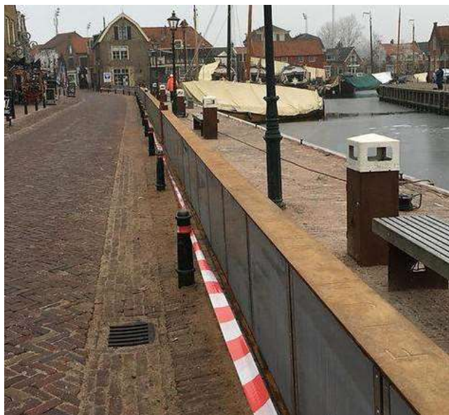
Figure 7-3: Hydrostatic Barrier (Flood Proofing, 2023)
