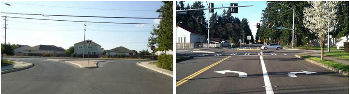
Figure 20. Sample Application of Forced Turn Island 30, 31
