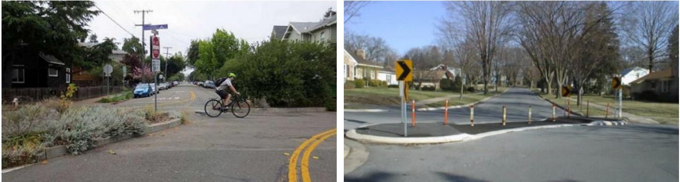
Figure 18. Sample Application of Diagonal Diverter 27, 28
