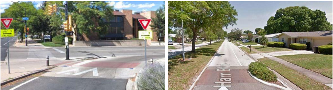
Figure 7. Sample Application of Speed Table 10,11
