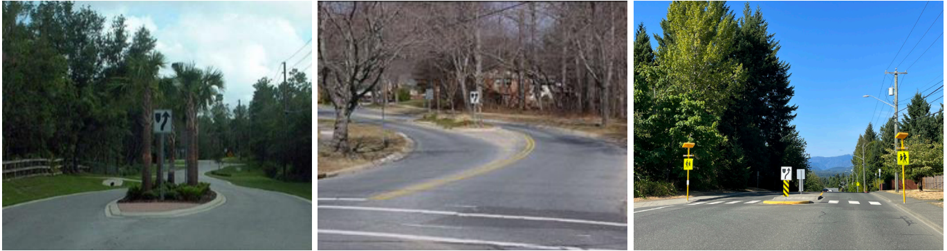
Figure 13. Sample Application of Median Island (Mid-Block – Left, Neighbourhood Entrance – Middle, With Crosswalk – Right) 20, 21
