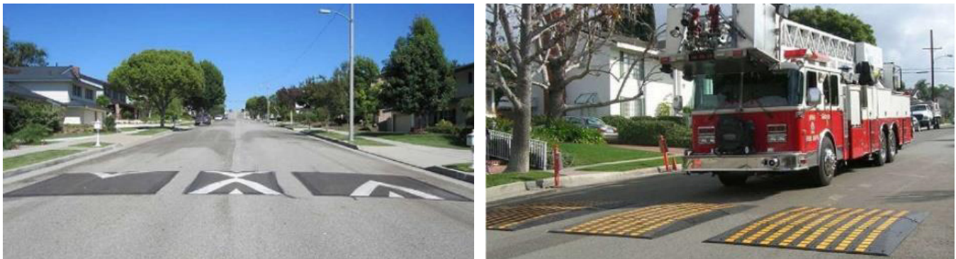
Figure 8. Sample Application of Speed Cushion 12
