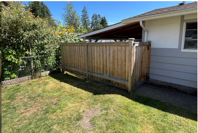
Figure 5: Existing fence screening along northeast side.
