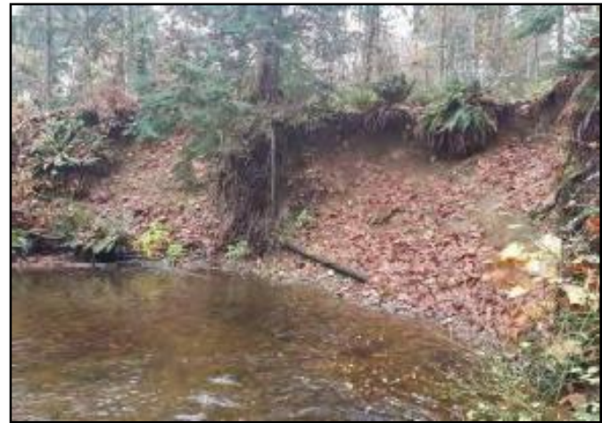
Degraded riparian corridor, creek bank requires stabilization
