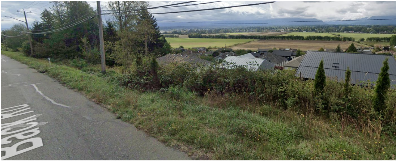
Figure 6: Example of a Back Road Segment without Guardrail Installed
