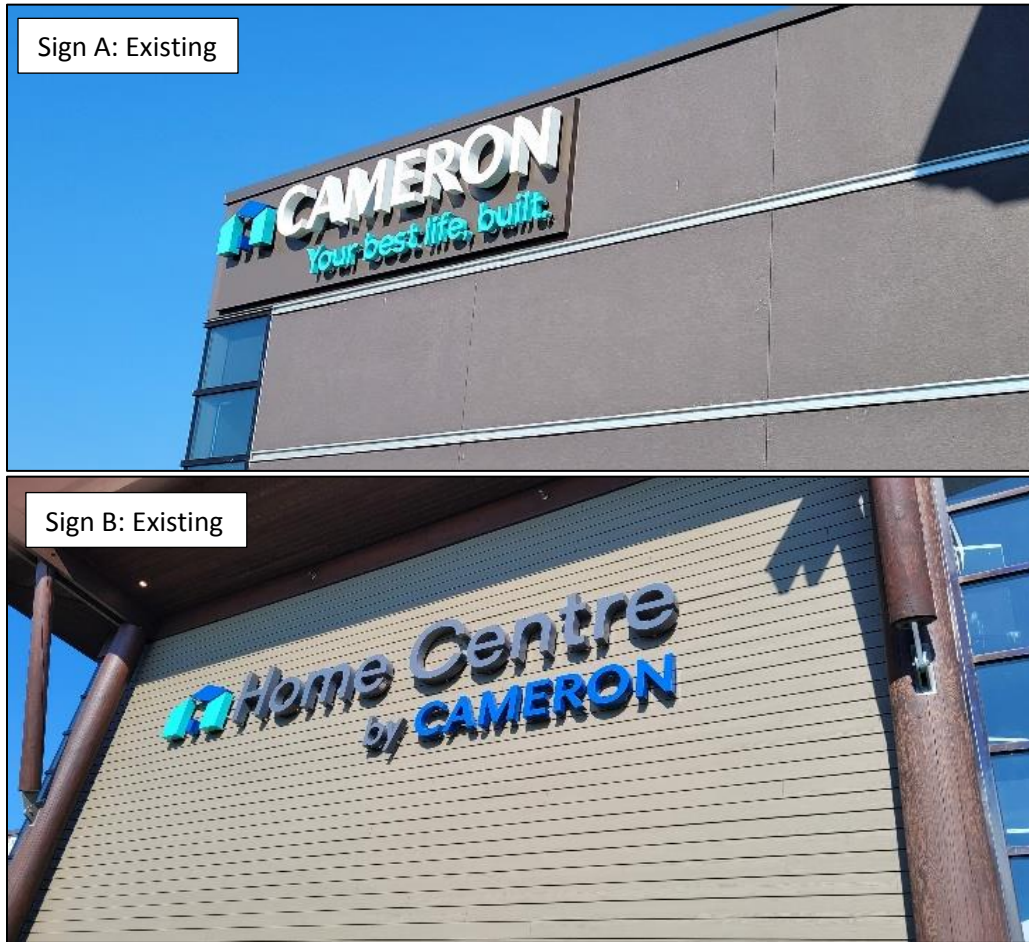
Figure 2: Existing Signage on South Building Face
